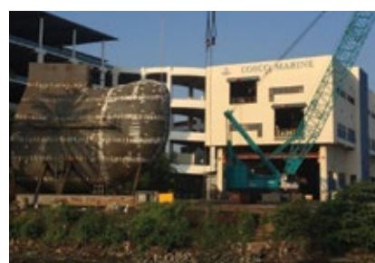
Ship Repair and Marine Engineering
